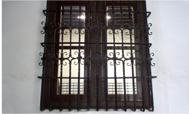
Ventana exterior enrejada
